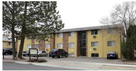
3635 Michigan Ave. Colorado Springs, CO 80910 #4
